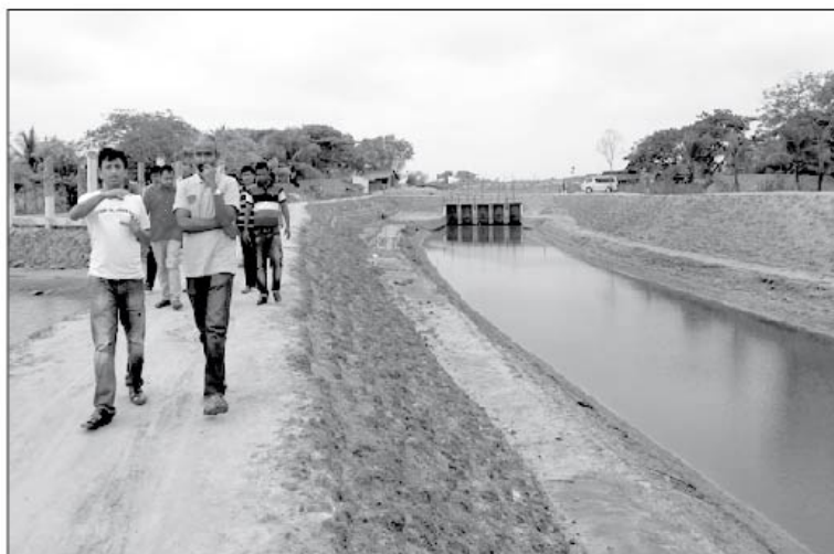
Canal re-excavation for water supply, irrigation and solve the water logging problem
