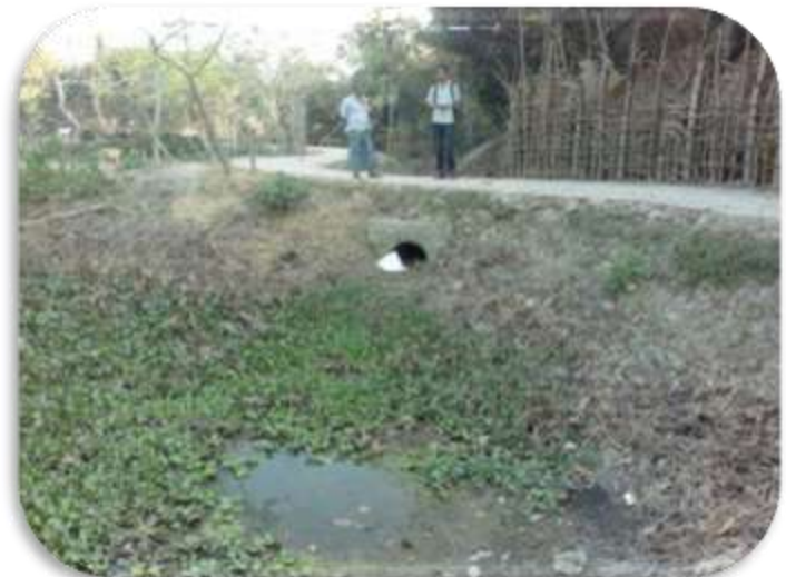
Inlet-outlet pipe and canal
