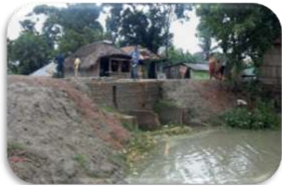
Picture: Gate becomes useless near Mathabanga
