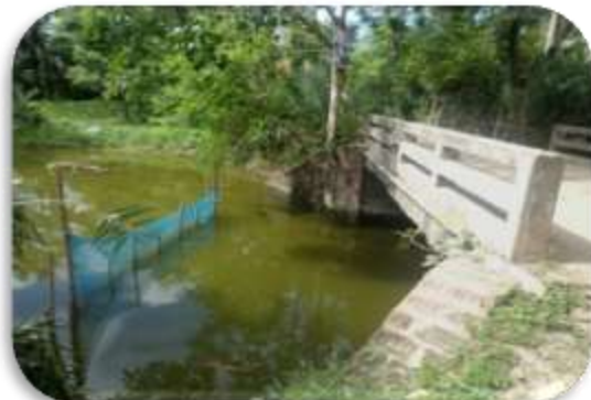
Picture: Rangemari canal become motionless due to blocked
